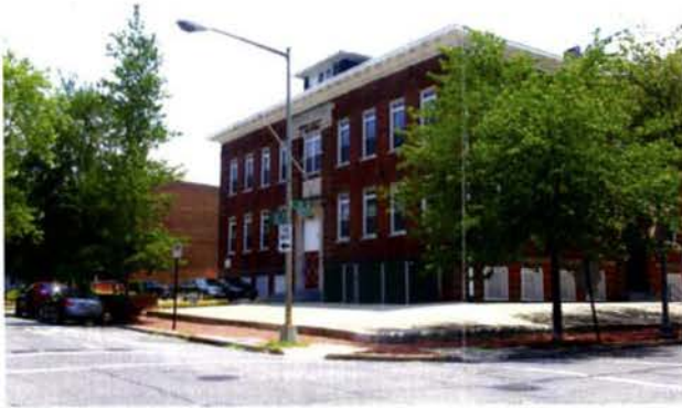
North Elevation Before
