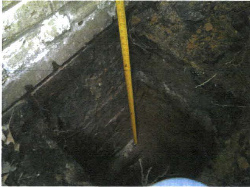
Wall Footing (Showing Depth)
