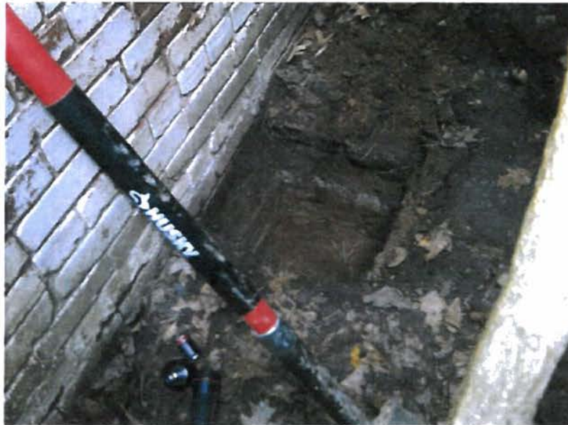
Test Pit Excavation
