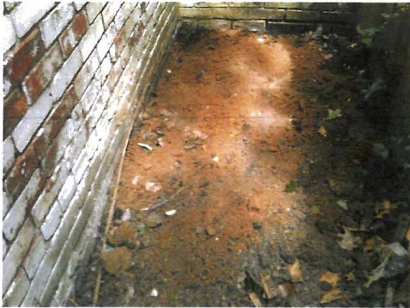
Test Pit Location
