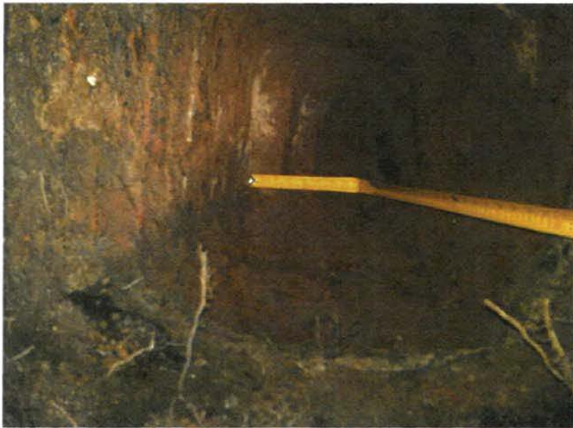
Wall Footing (Showing Width)
