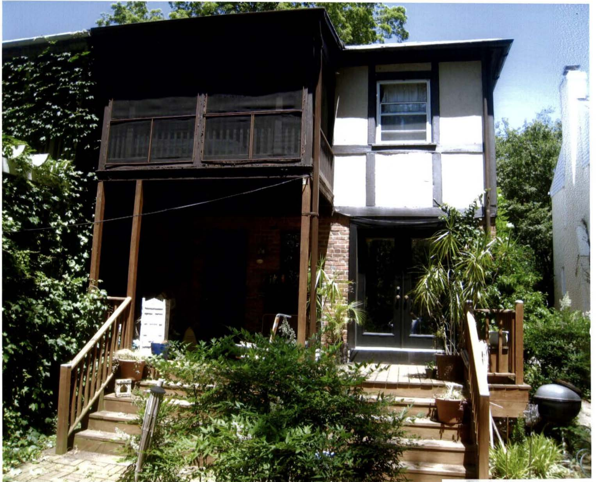
View of Rear Yard and South Facade
