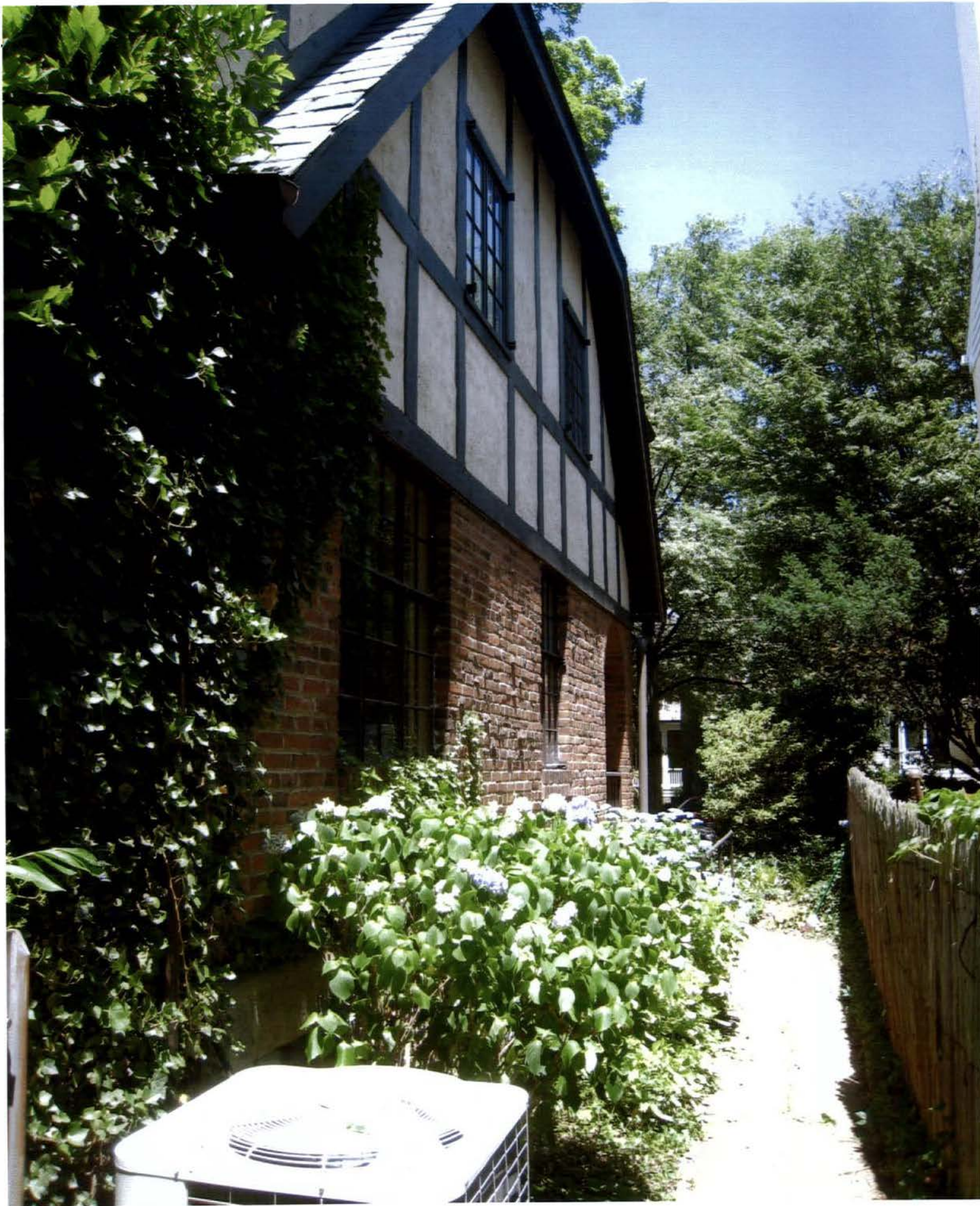
View of Side Yard and East Facade
