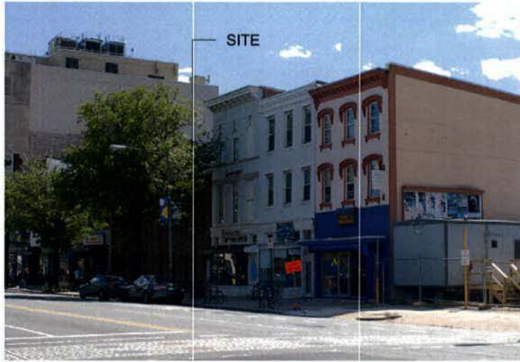
① 14TH STREET (LOOKING SOUTHWEST)
