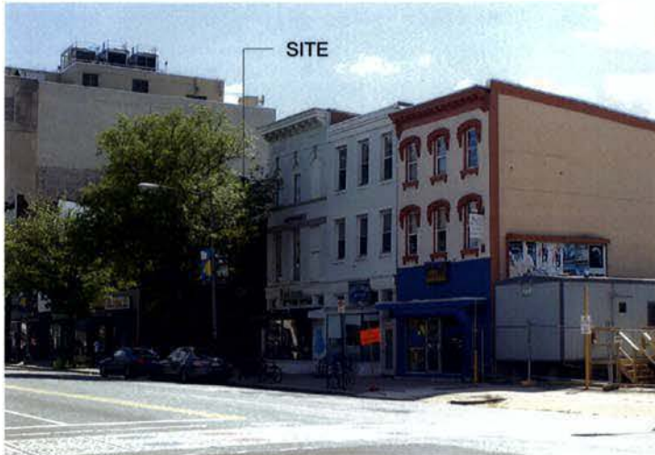
① 14TH STREET (LOOKING SOUTHWEST)
