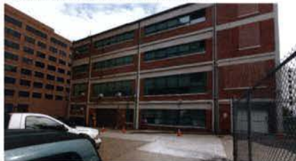
27. View of SQ 50 from project site
