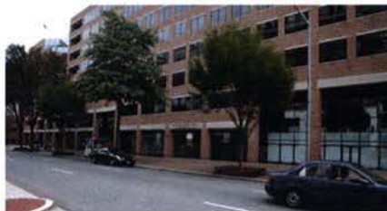
21. View NE towards SQ 50 from 23rd ST NW
