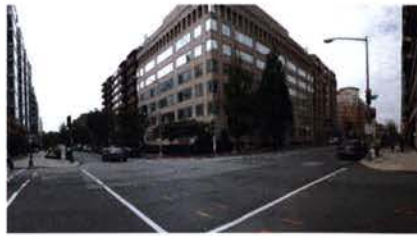
2. View SW toward SQ 37 from corner of 23rd & M ST NW
