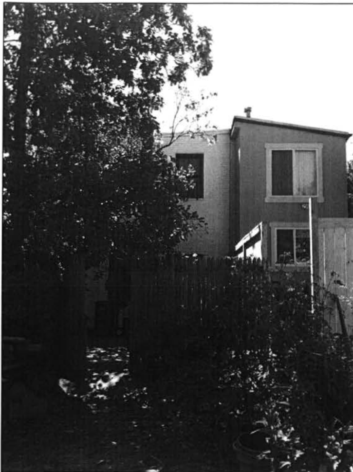
2 REAR OF HOUSE C-4
