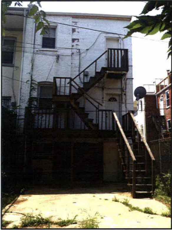
REAR OF PROPERTY FROM REAR ALLEY
