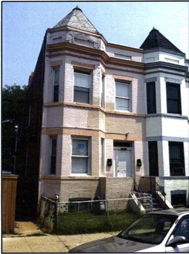
FRONT OF PROPERTY FROM OTIS PLACE
