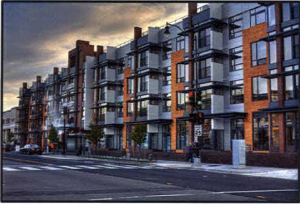
ALLEGRO APARTMENTS 3460 14th Street NW 297 Units
