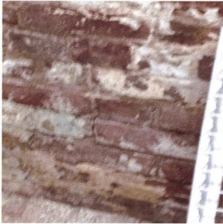
Fig. 3: Left Wall of Basement @ Rear of House
