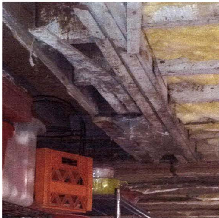
Fig. 8: First Floor Framing @ Stair Opening
