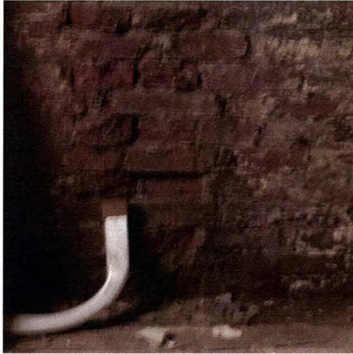
Fig. 5: Left Wall of Basement @ Rear of House
