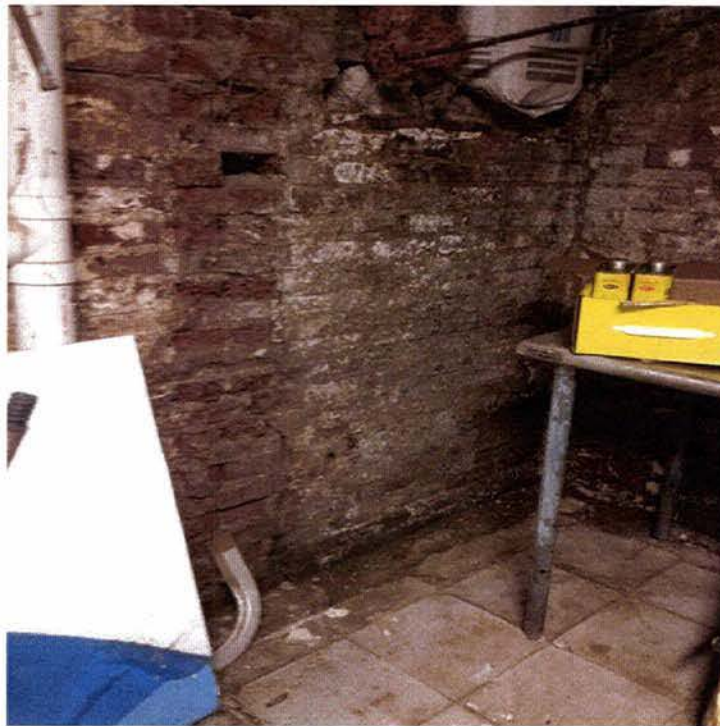
Fig. 4: Left Wall of Basement @ Rear of House
