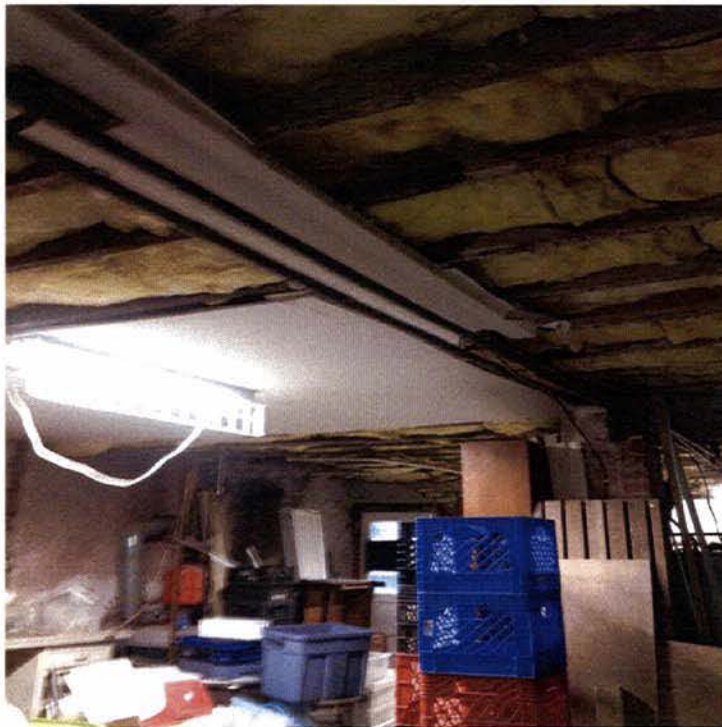
Fig. 6: Steel Beam @ First Floor Framing is removed
