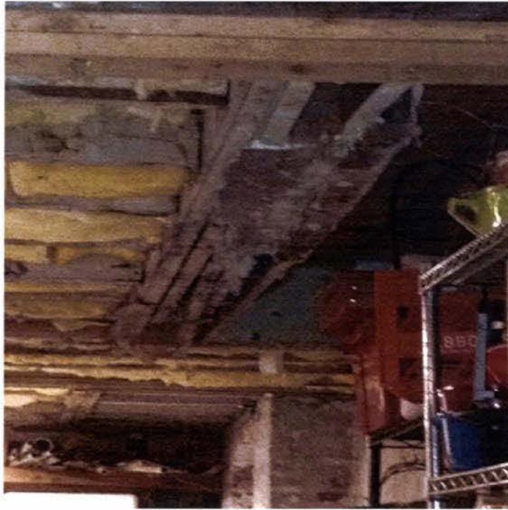
Fig. 7: First Floor Framing @ Stair Opening
