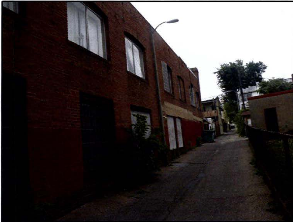
WEST SIDE OF PROPERTY FROM ALLEY
