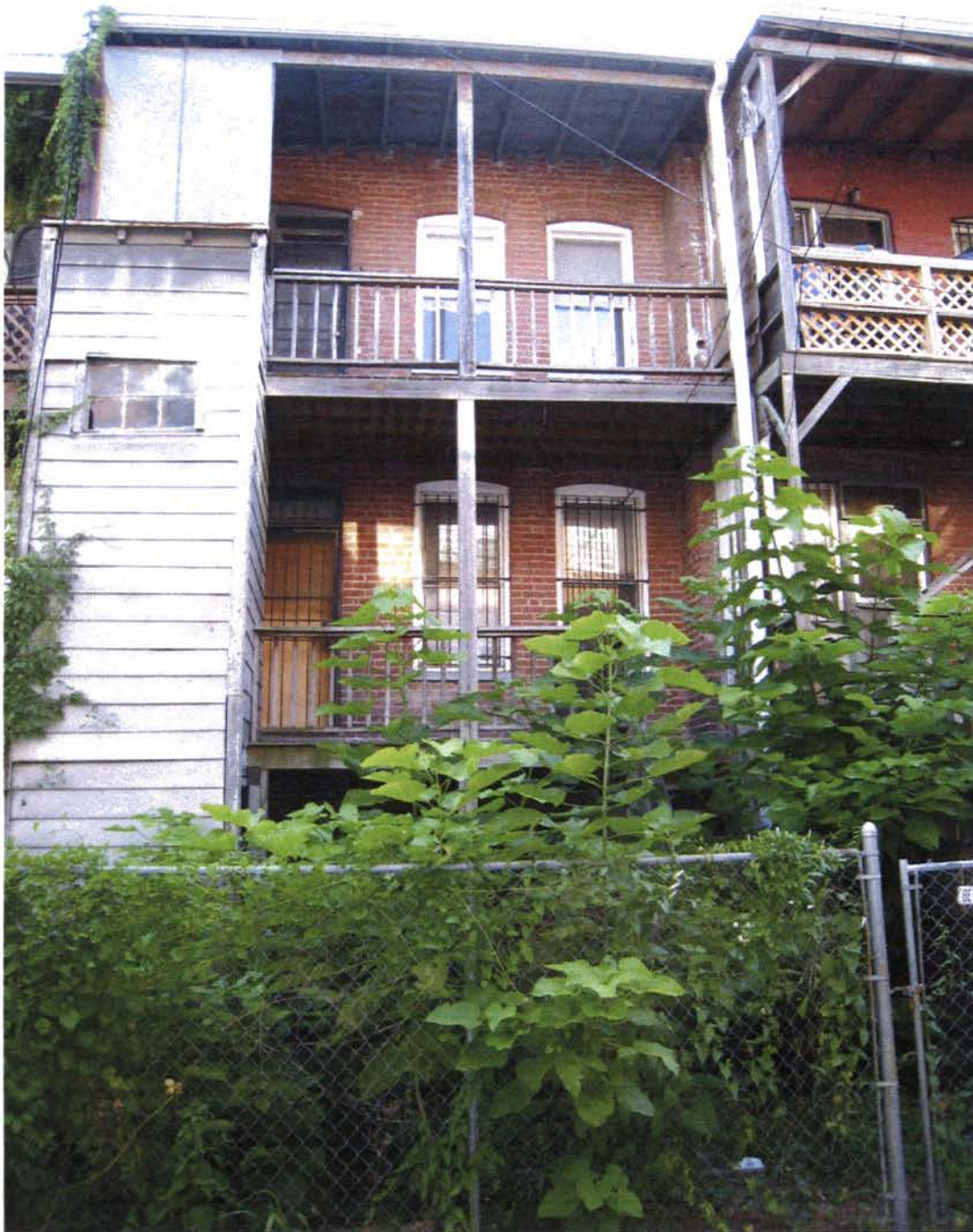
Fig. 10. Alley façade (facing east).
