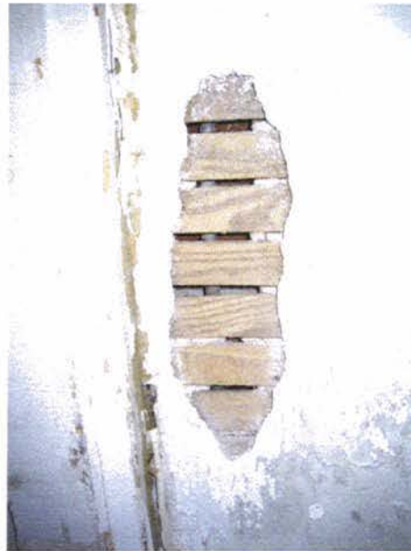
Fig. 4. Original plaster on lath throughout.
