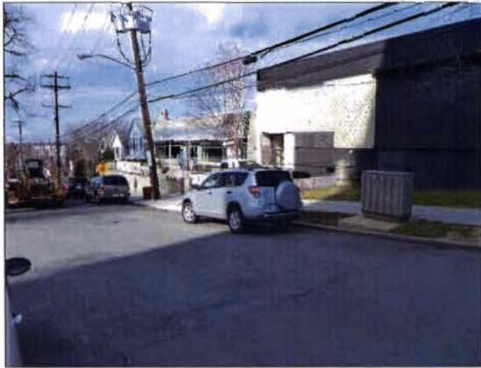
① P1 VIEW OF FRONT FACADE FROM BRANDYWINE ST.
