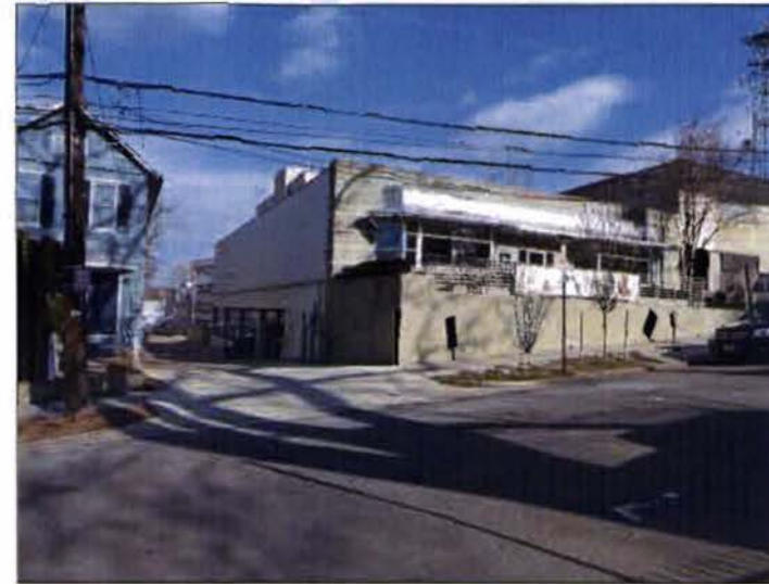
② P1 VIEW OF FRONT / ALLEY FACADES FROM BRANDYWINE ST.
