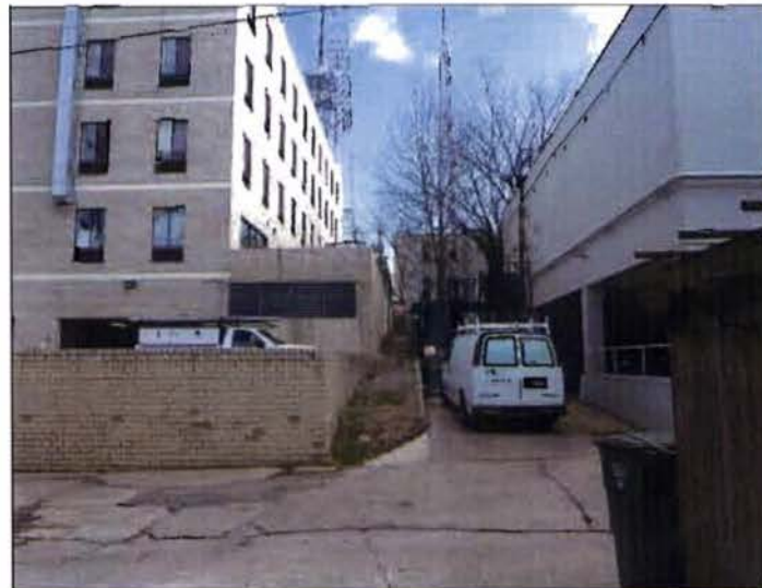
③ P1 VIEW OF REAR FACADE FROM ALLEY
