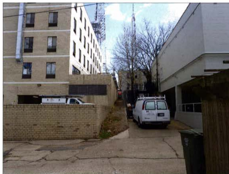
③ VIEW OF REAR FACADE FROM ALLEY P-1
