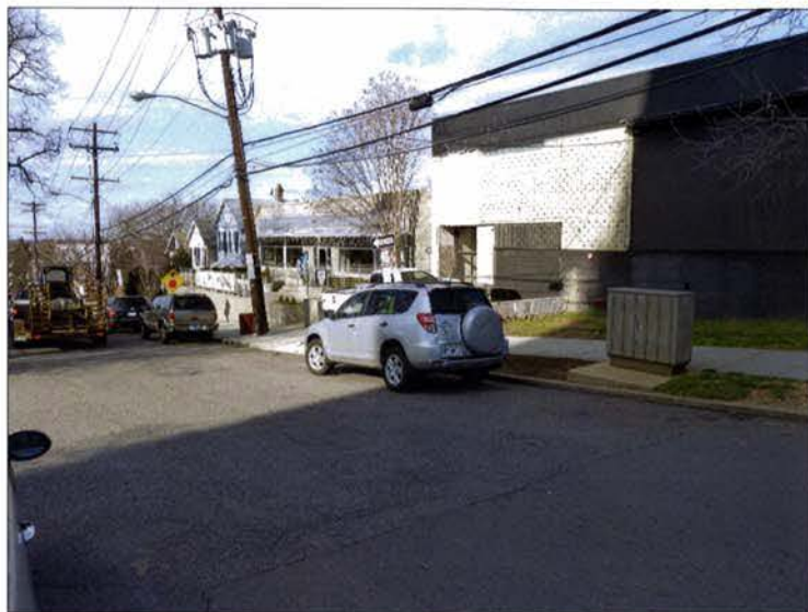
① VIEW OF FRONT FACADE FROM BRANDYWINE ST. P-1
