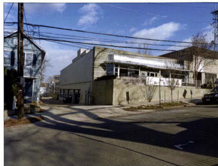
② VIEW OF FRONT / ALLEY FACADES FROM BRANDYWINE ST. P-1
