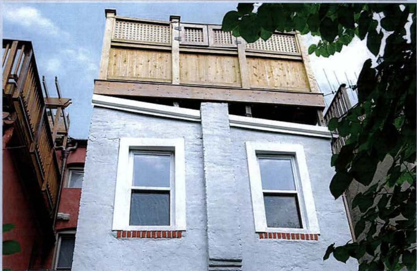
ROOF TOP DECK
