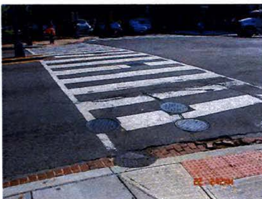
North Capitol Street/K Street – Northwest Corner
