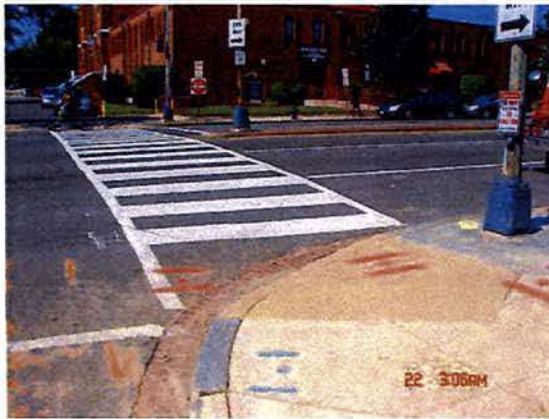
North Capitol Street/L Street –Northeast Corner
