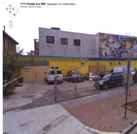
View from North
