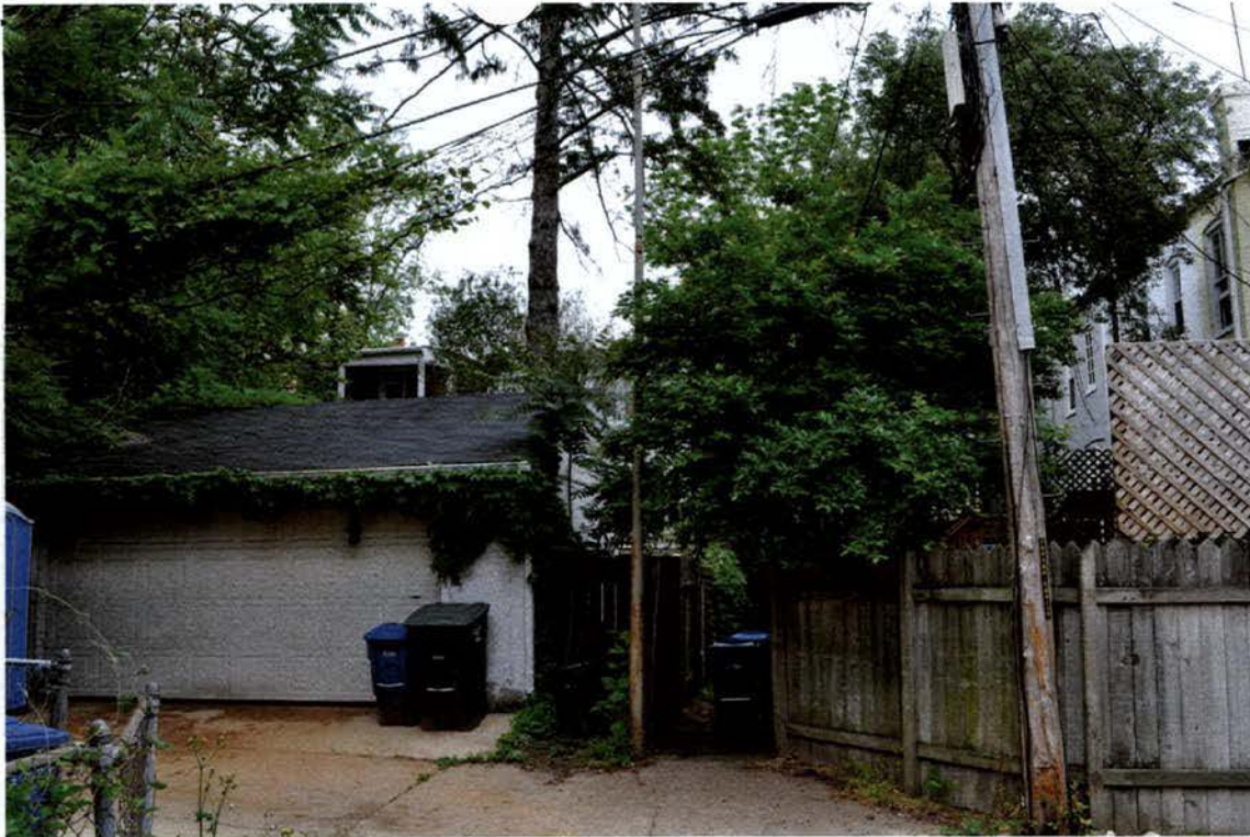
Rear View of Subject Property from West (Alley)
