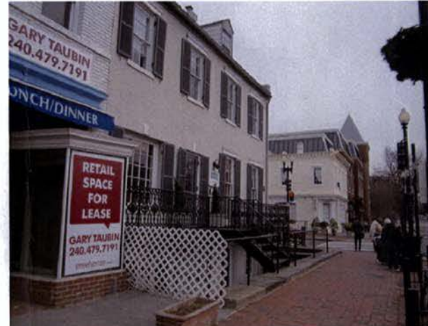
4 EXISTING EXTERIOR STOREFRONT
