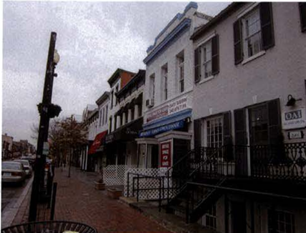
3 EXISTING EXTERIOR STOREFRONT
