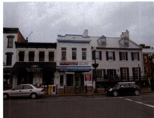
2 EXISTING EXTERIOR STOREFRONT
