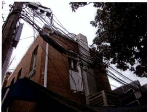
3 EXISTING EXTERIOR REAR
