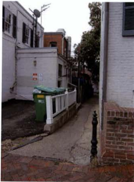
1 EXISTING EXTERIOR REAR FROM 28TH STREET, NW
