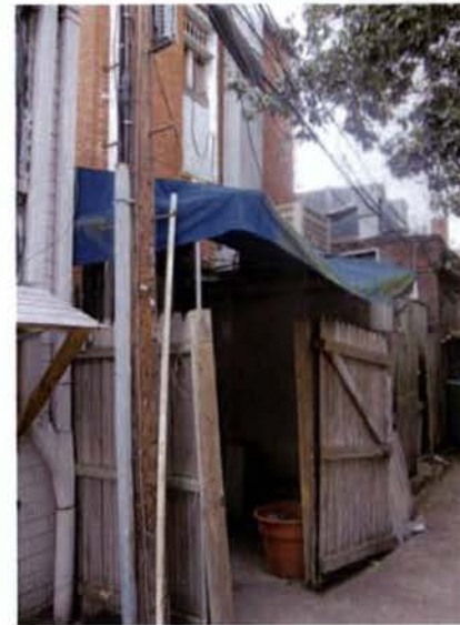
2 EXISTING EXTERIOR REAR
