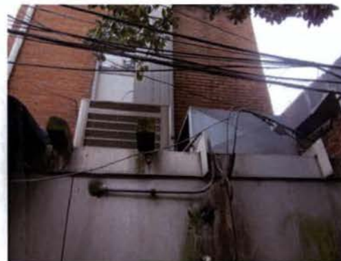
4 EXISTING EXTERIOR REAR
