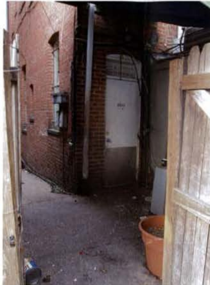
1 EXISTING EXTERIOR REAR
