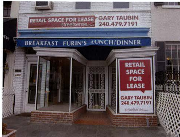
1 EXISTING EXTERIOR STOREFRONT
