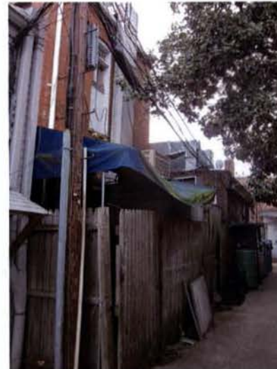
4 EXISTING PHOTO EXTERIOR ELEVATION (REAR)
