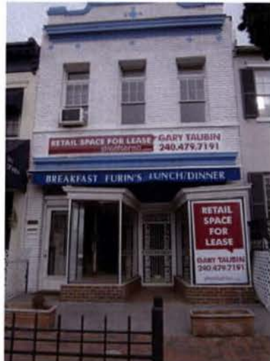
3 EXISTING PHOTO EXTERIOR ELEVATION (FRONT)
