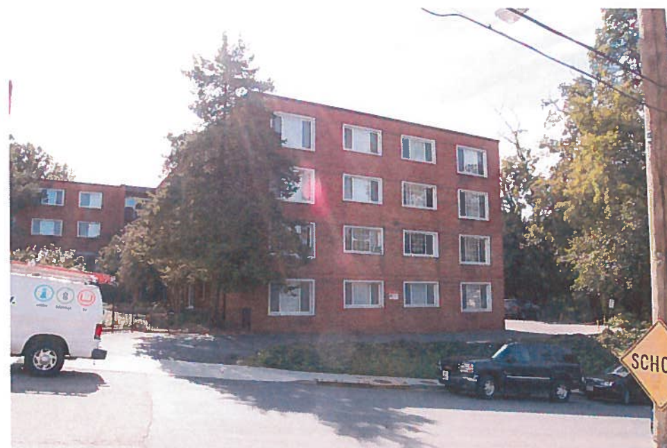
adjacent apartments to east on rock creek ford road
