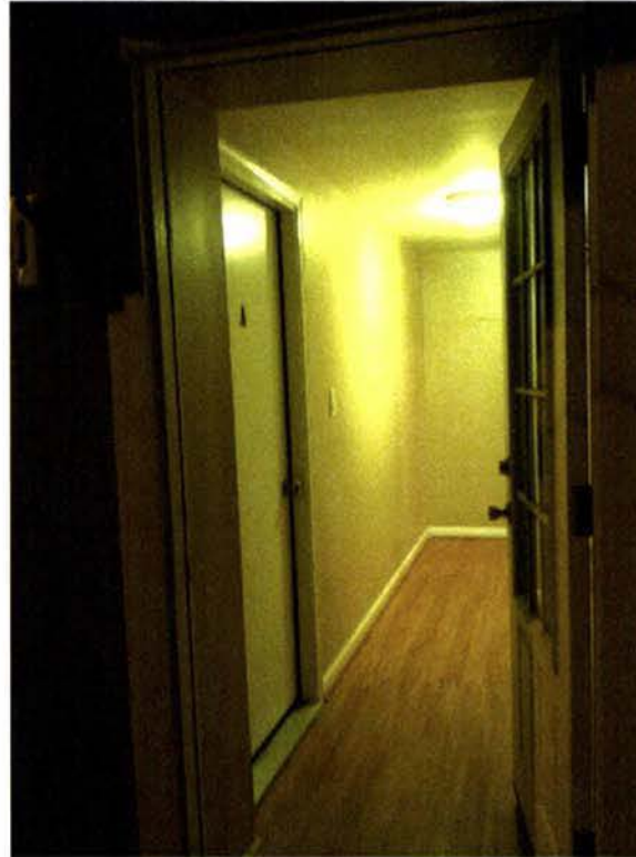
Front Door Entry, Unit A on Left
