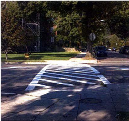
16 th Street/Crittenden Street (looking west)
