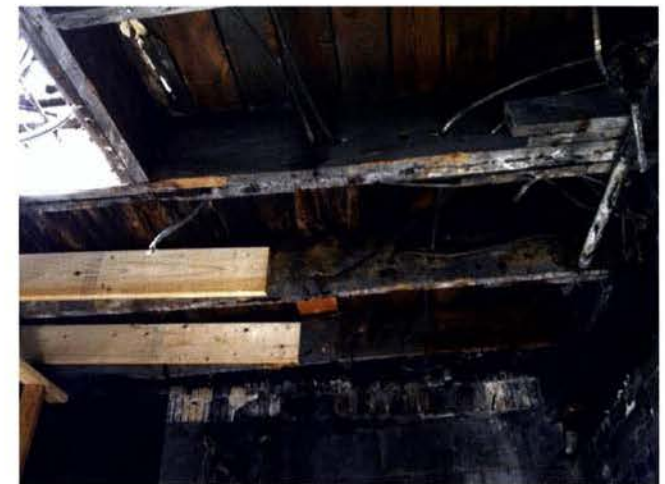
View of the roof structure
