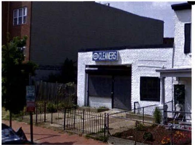
View of the R Street facade
