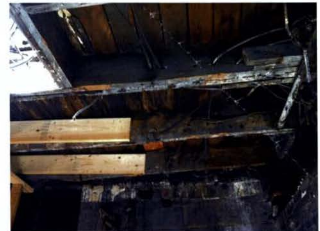
View of the roof structure
