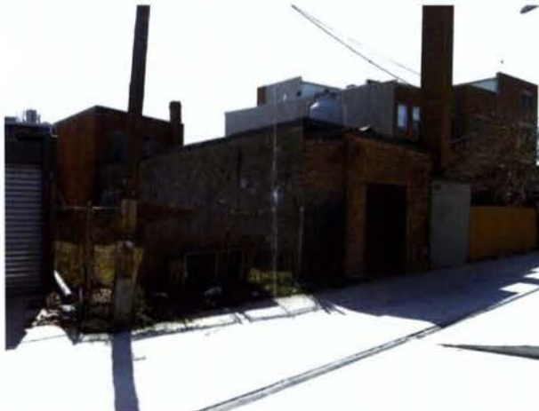
View of the rear of the property
