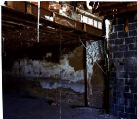
View inside the structure
