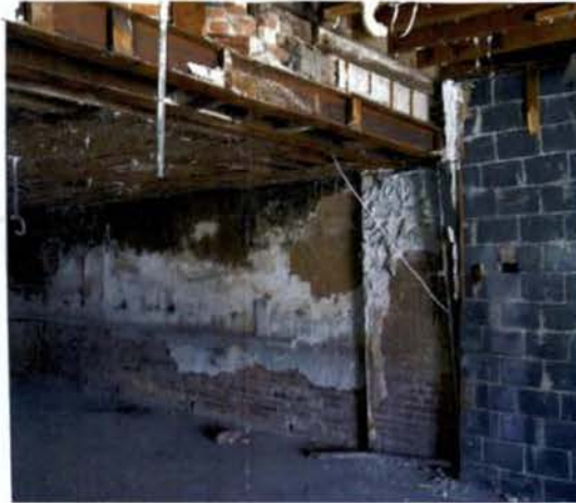
View inside the structure
