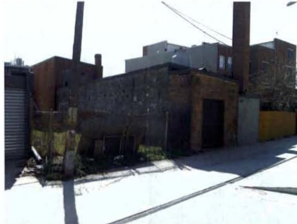
View of the rear of the property
