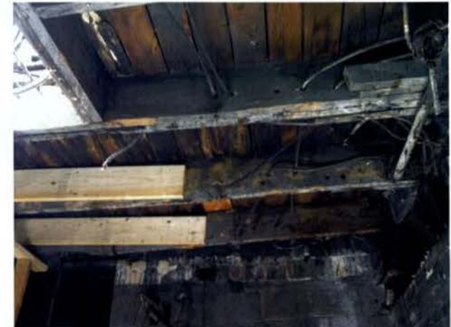
View of the roof structure
