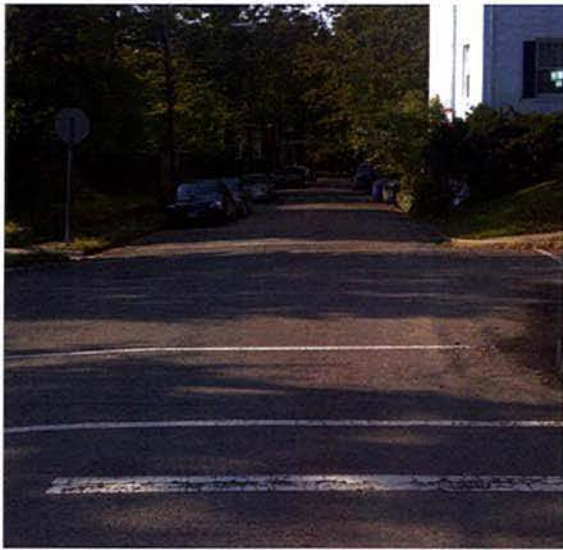
Piney Branch Avenue/Crittenden Street (looking north)
