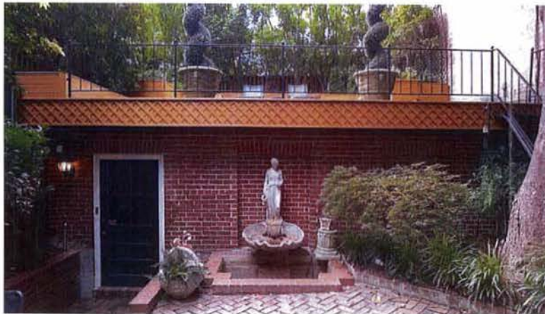
Garage Courtyard Facade & Roof Deck
