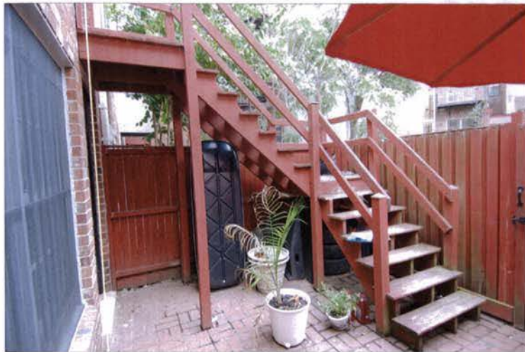
1 Photo of Existing Deck (to be removed and replaced) from rear Yard A-7 N.T.S.
