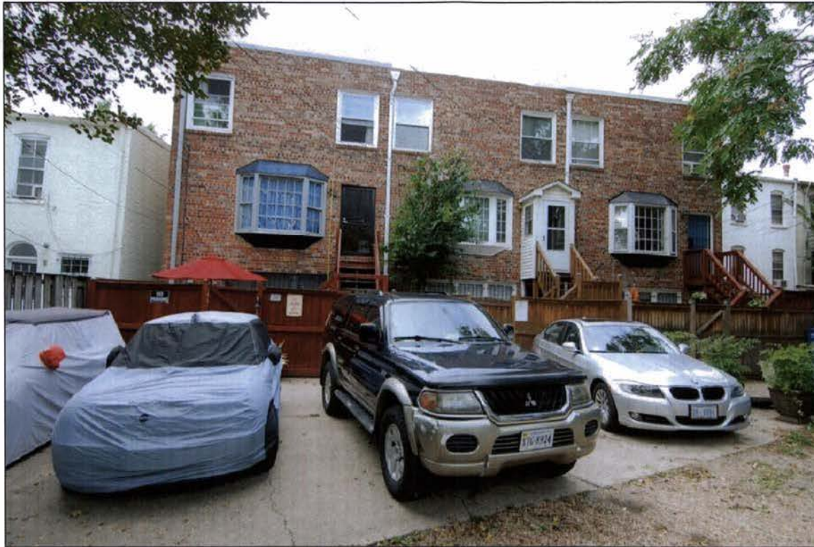
1 Photo of Existing looking North from Alley A-7 N.T.S.
