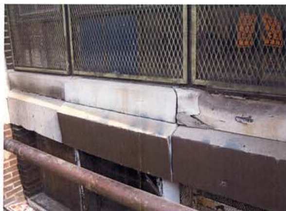
Existing concrete sill at front elevation.
