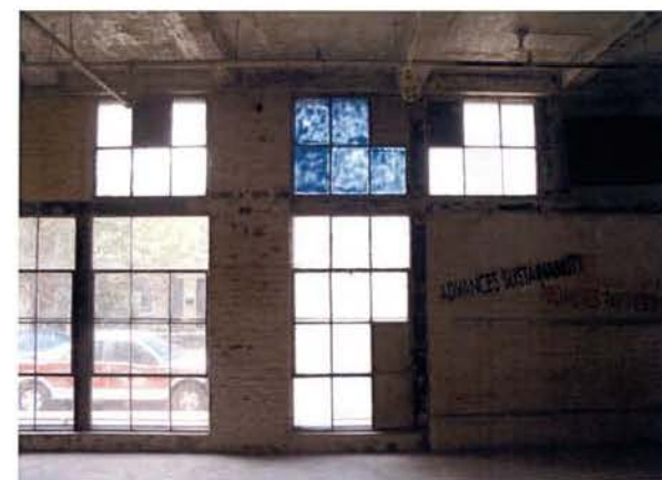
Existing window configuration.
