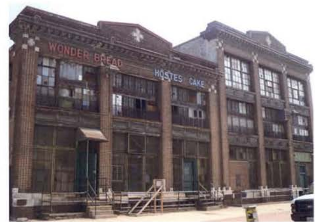
S Street Facade, looking NE
