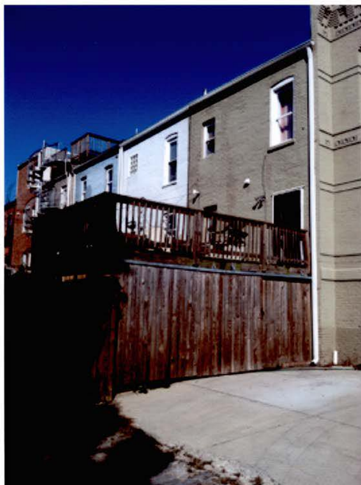
VIEW FROM ALLEY, LOOKING WEST
