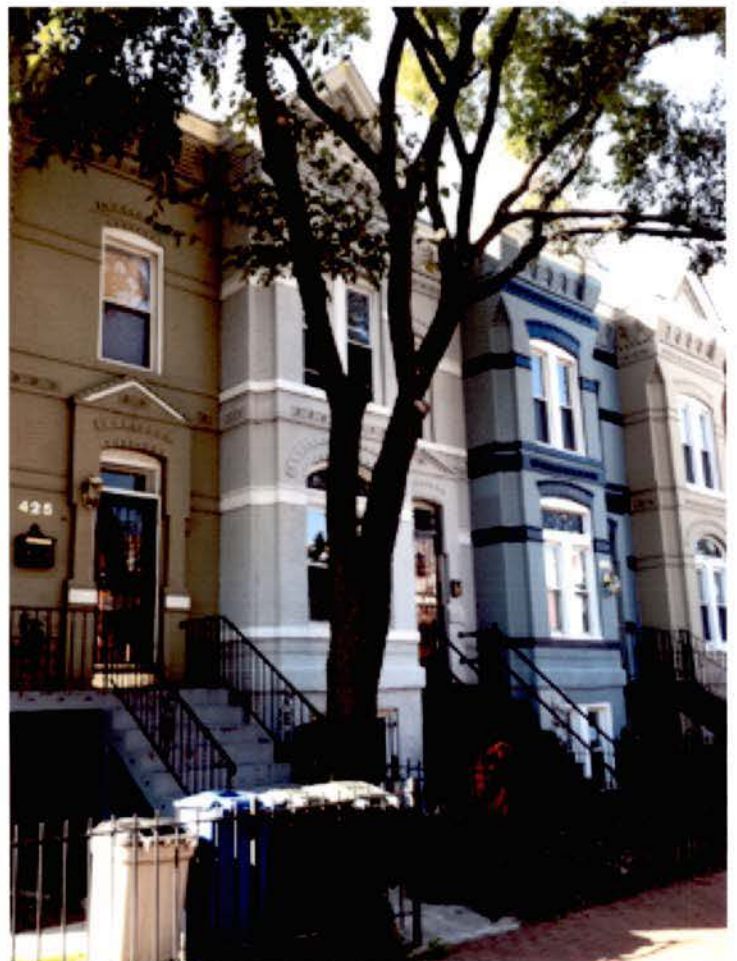
VIEW FROM M STREET, LOOKING WEST
