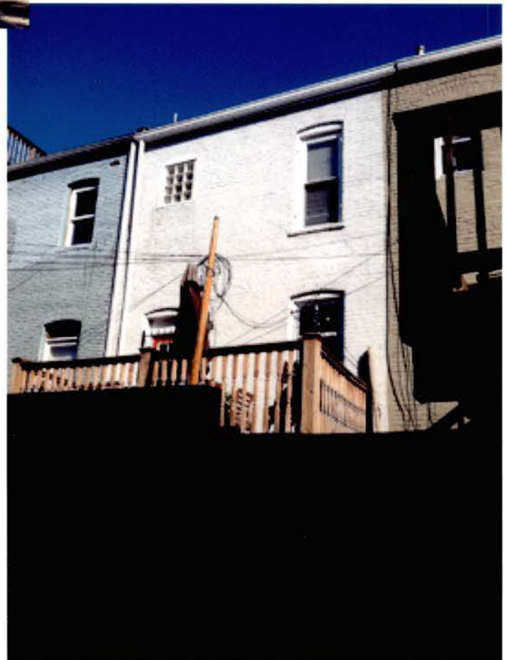
REAR OF HOUSE, 423 M STREET NE
