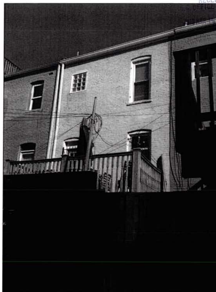
2 REAR OF HOUSE C-4
