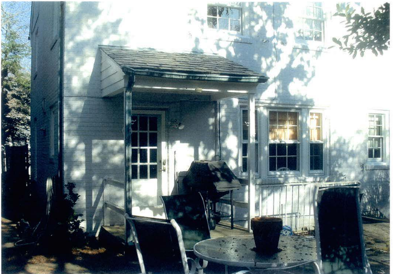
Existing area for Addition
