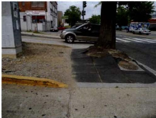
Figure 1: Example of narrow, non ADA-compliant sidewalk along Rhode Island Avenue
