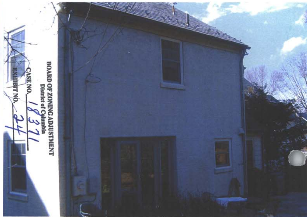
EAST, ADDITION LOCATED TO RIGHT OF FR DRs ②
