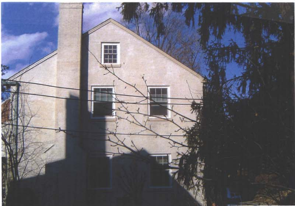
SOUTH, ADDITION LOCATED BEHIND HOUSE TO RIGHT ③
