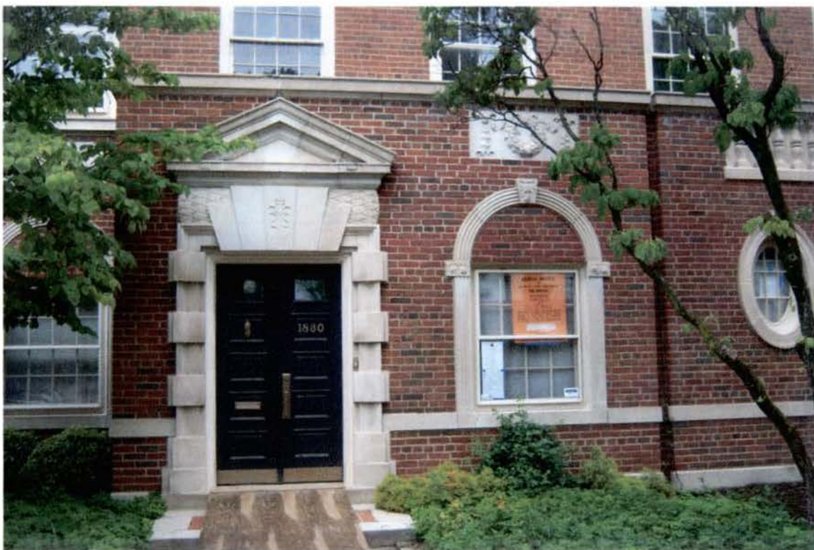
① AS SEEN FROM 24 th STREET, NW.
