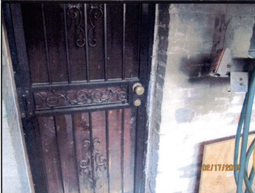
Picture of basement access
