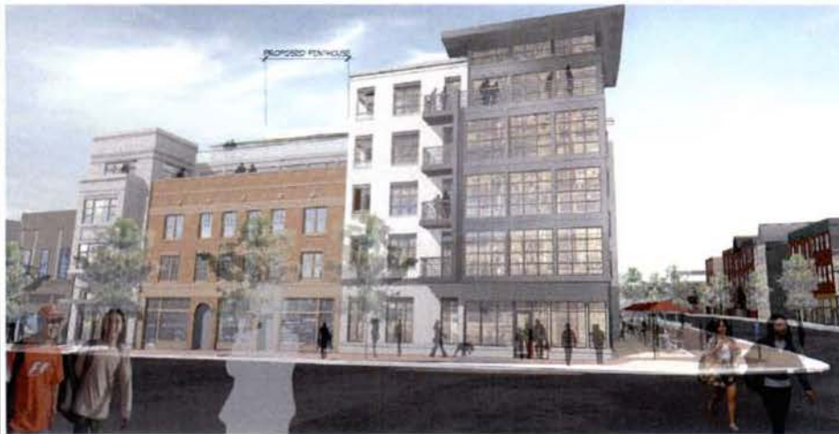
VIEW FROM THE INTERSECTION OF 9 TH STREET AND N STREET NW
