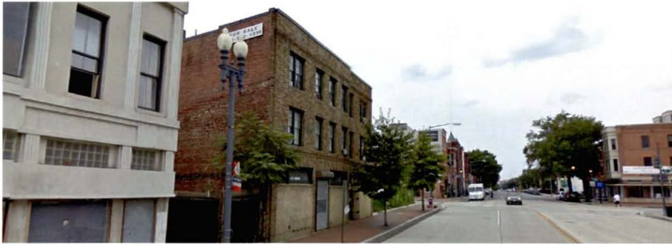
1. VIEW ALONG 9TH STREET, LOOKING NORTH
