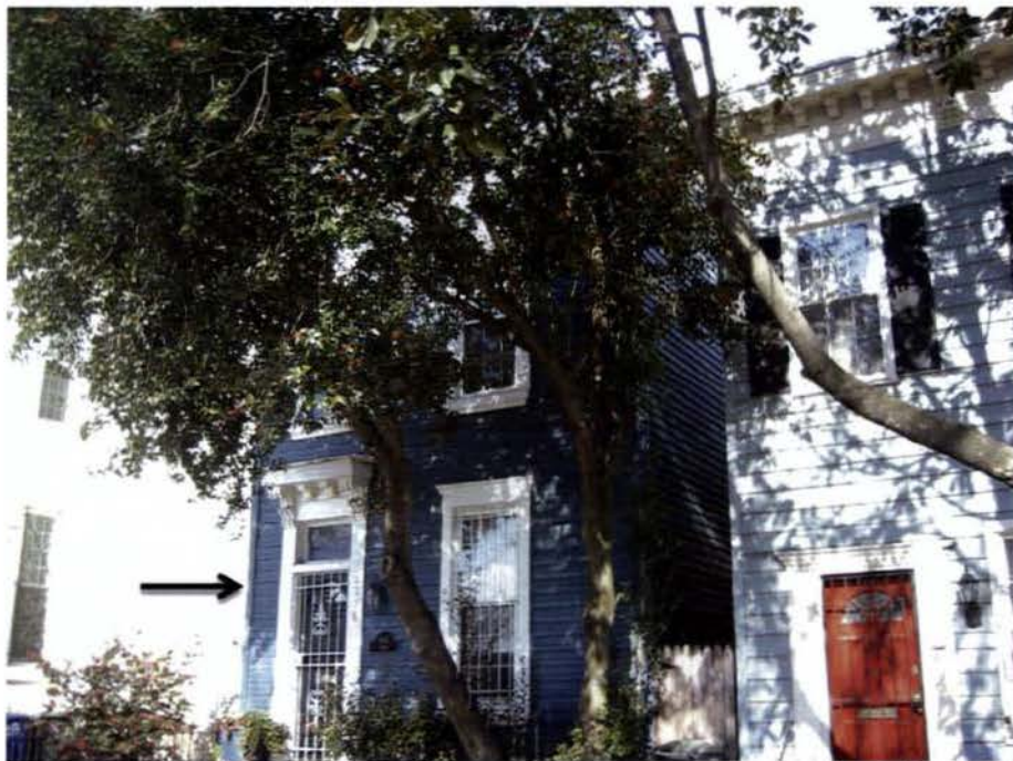
Front Corner View
