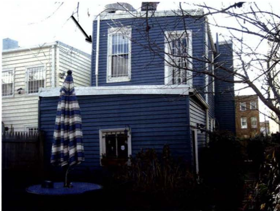
Rear Corner View
