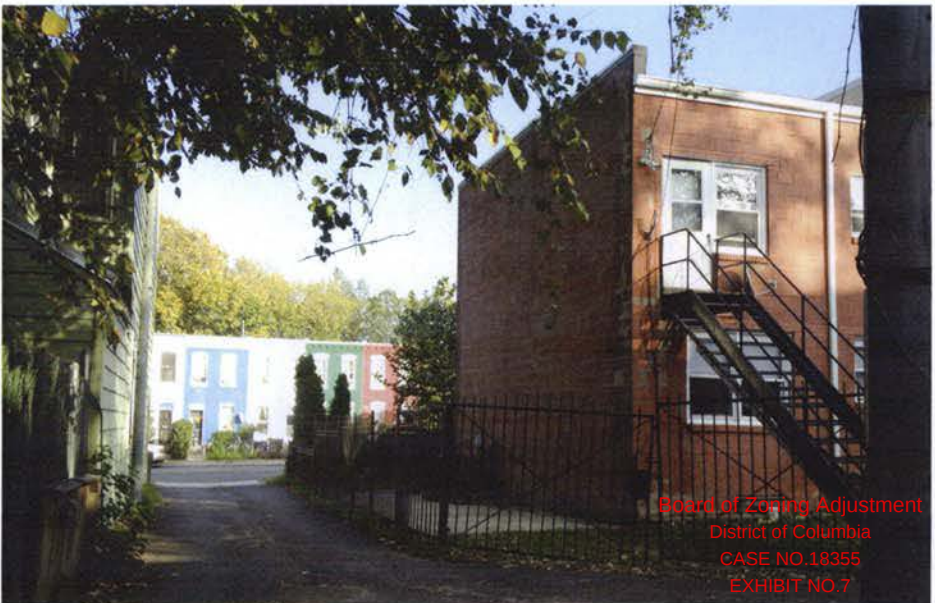
View from public alley facing Southeast
