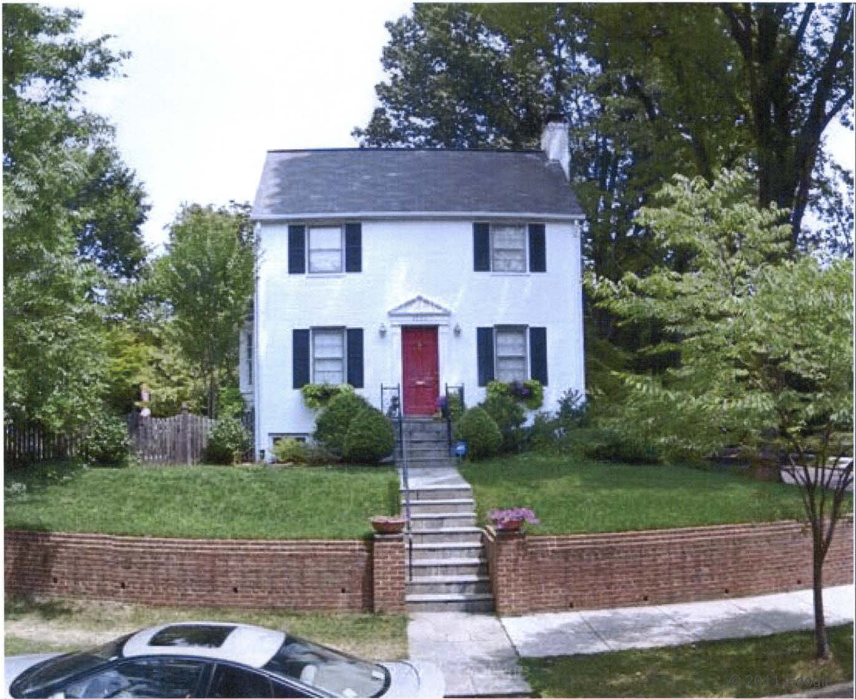
4225 45th Street NW (Property Directly Across the Street)
