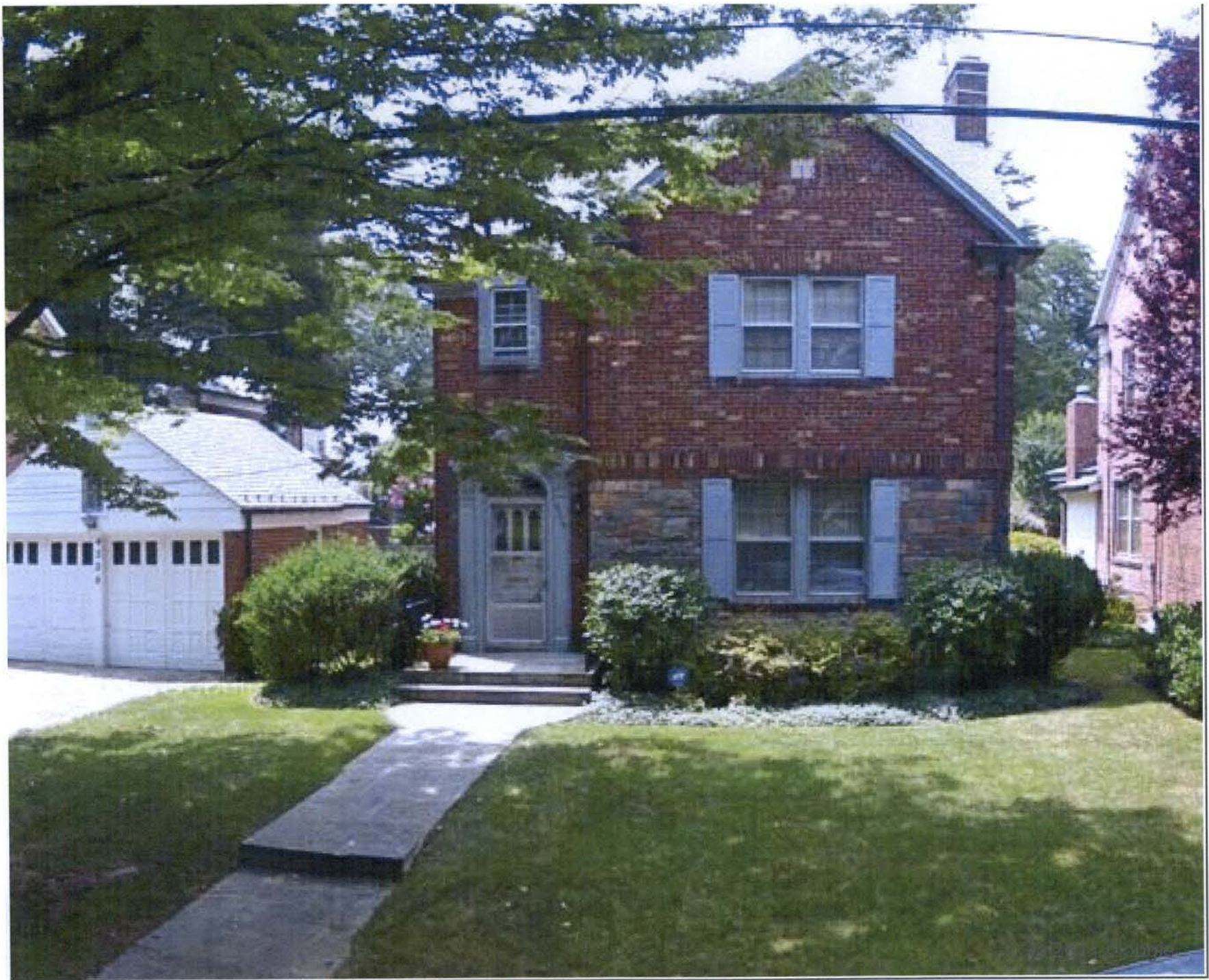
4224 45th Street NW (Adjoining Property to the North)
