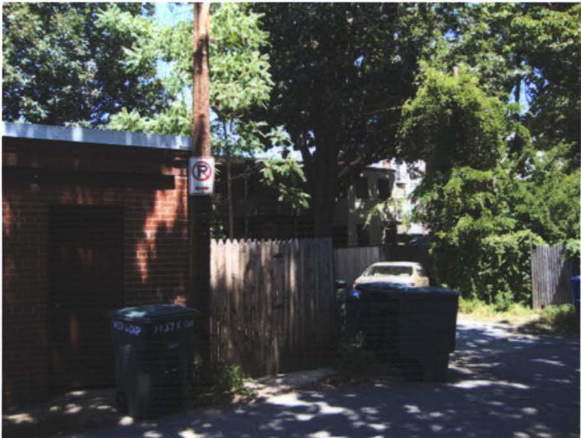
VIEW OF REAR FROM ALLEY, LOOKING EAST
