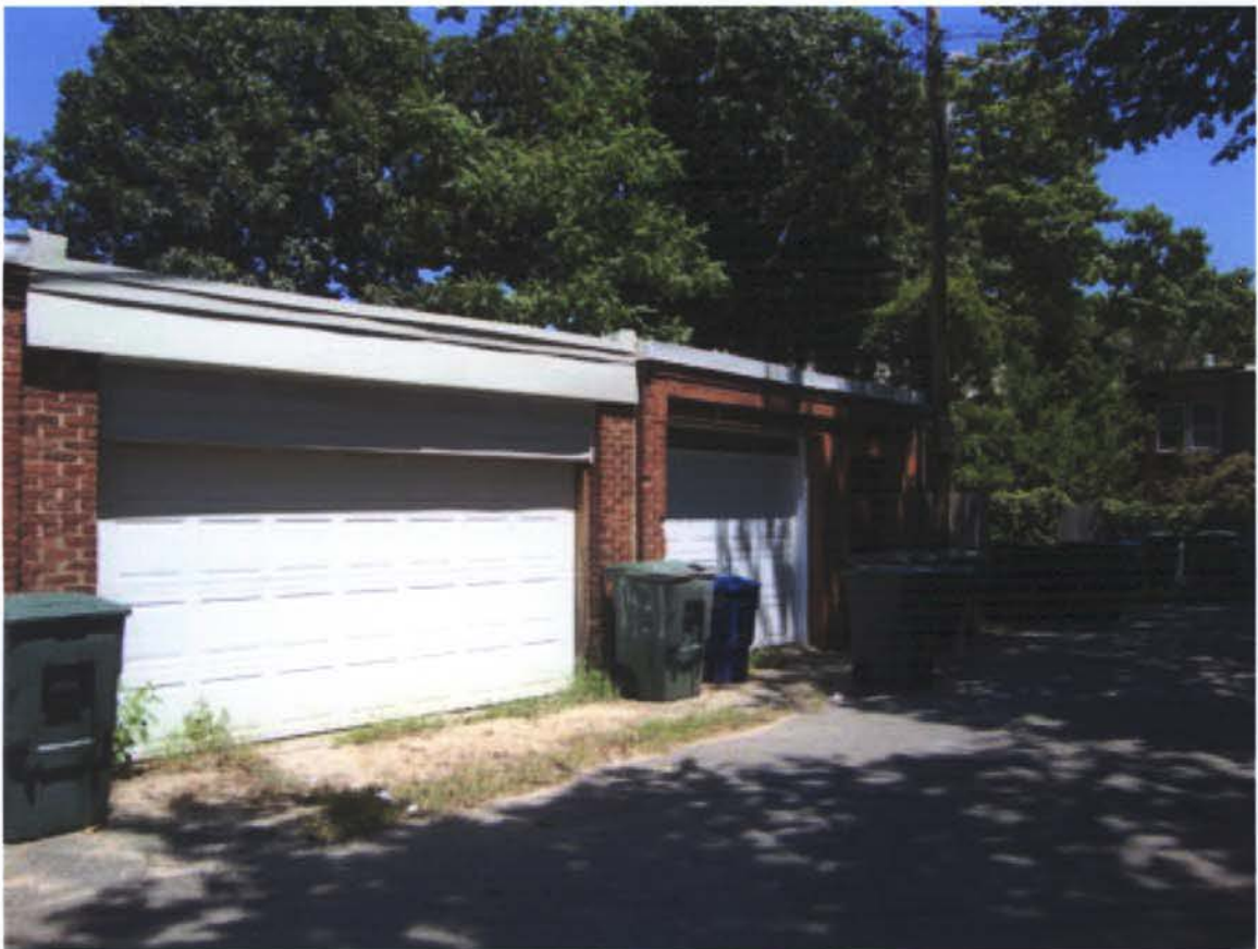
VIEW OF ALLEY, LOOKING EAST
