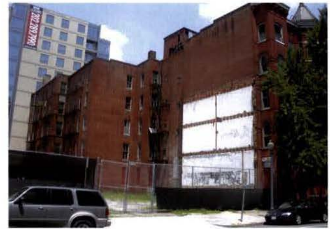
View Northeast from G Street NW
