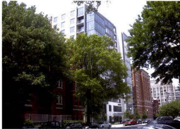
View North along 3rd Street NW
