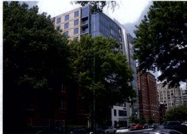
View North along 3rd Street NW
