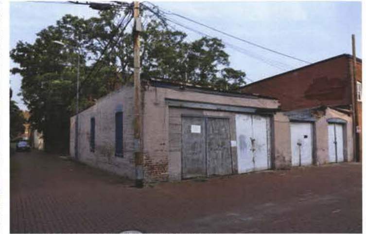
VIEW OF SITE - LOOKING SOUTHEAST
