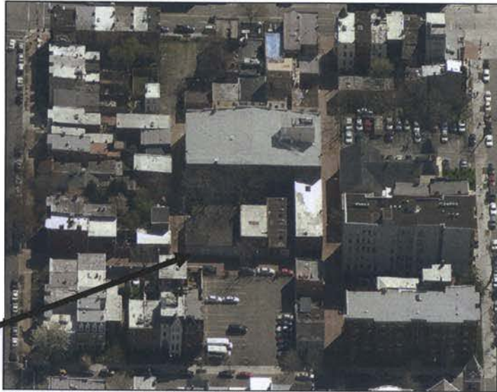
View of the Property (identified with an arrow) looking east across 10 th Street
