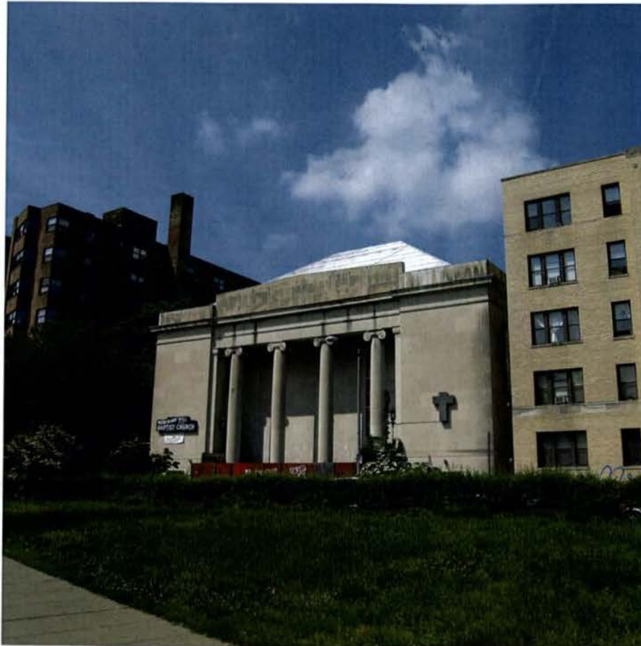
view of east facade of church from 16th Street
