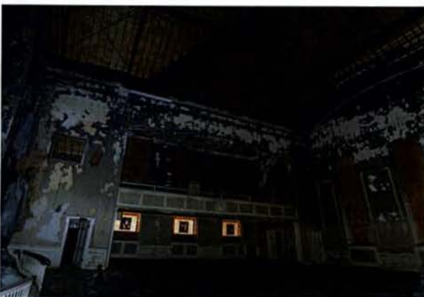
view of church interior showing damage from 2008 fire
