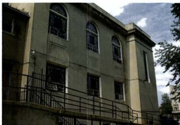
view of south facade of church
