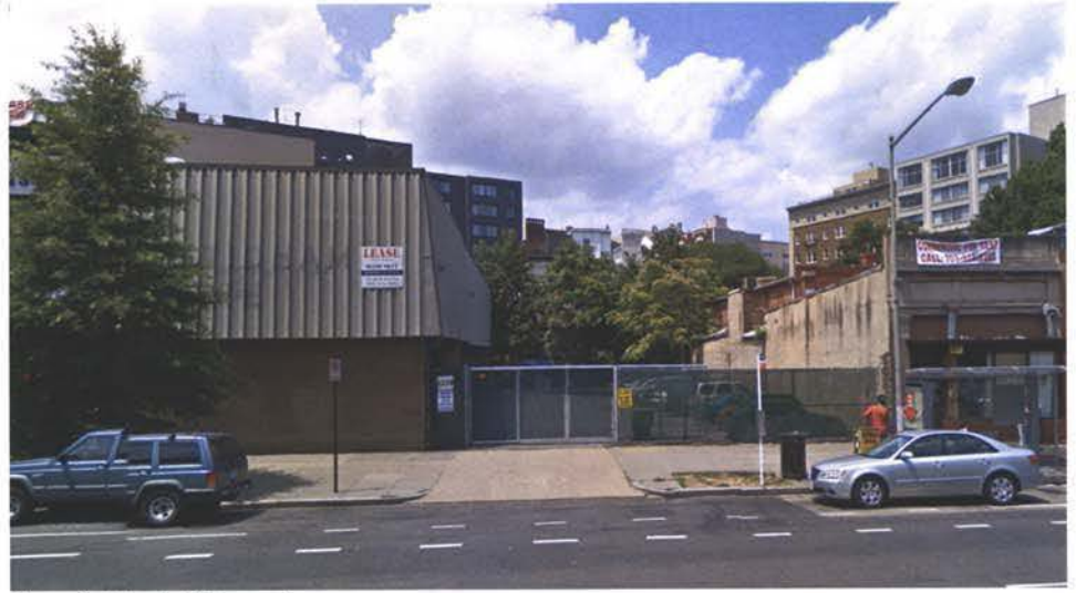
View of existing building on site
