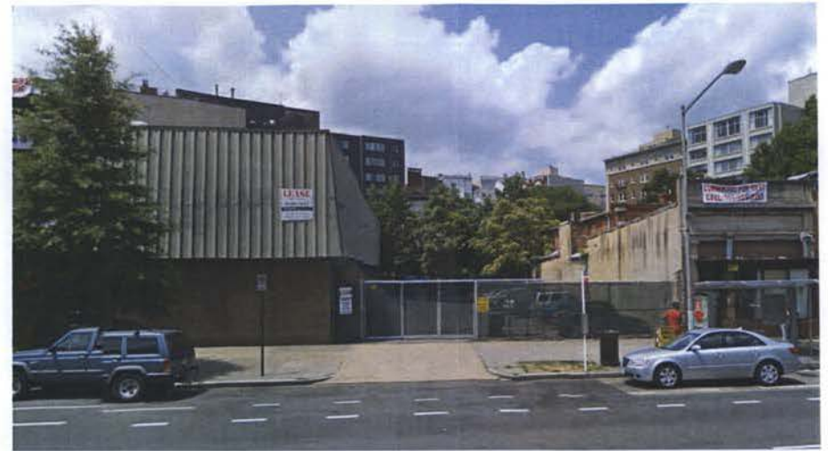
View of existing building on site
